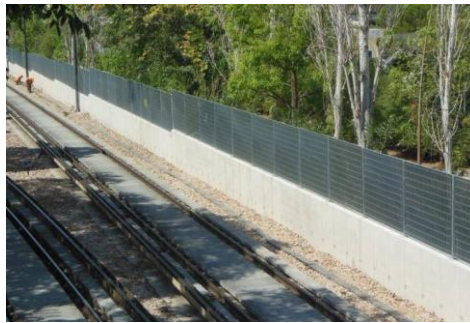
Figure 4.1 Noise barrier completed at Quiet Track test site in ISAP line 1
